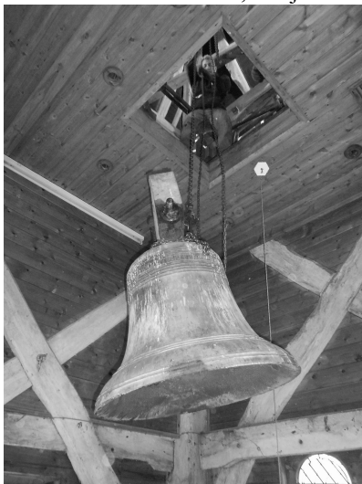
After several winches were used to get it out of its bell pit and across the frame, the Berrick Salome tenor is carefully lowered by Paul Lawrence
